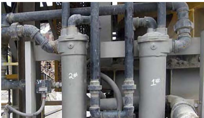
Model 816BC Flow Switch mounted on lube oil circuit for rock crusher at plant in Maryland.
